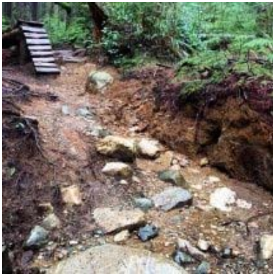
Floppy Bunny Trail erosion. Larger photo below...
